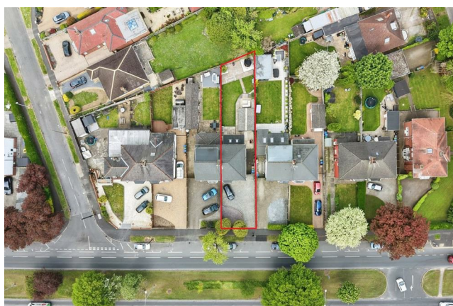
Aerial view of the property
